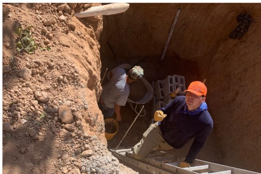
INSTALLING A WATER SYSTEM
