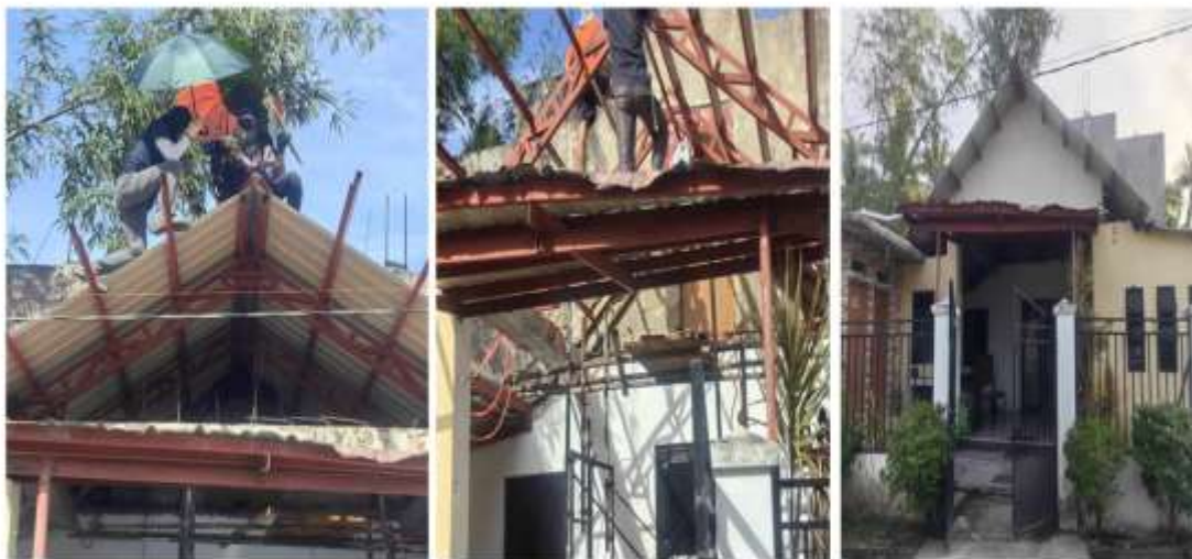
REPAIRS AND RENOVATIONS
